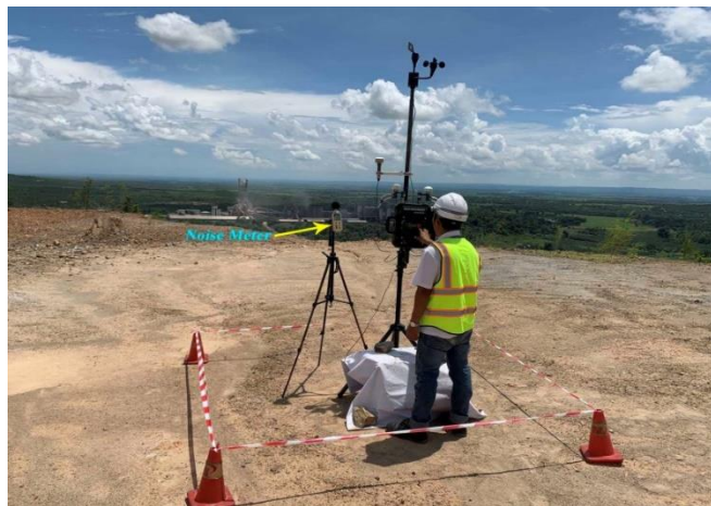
Figure-34: Measuring noise level at project site
