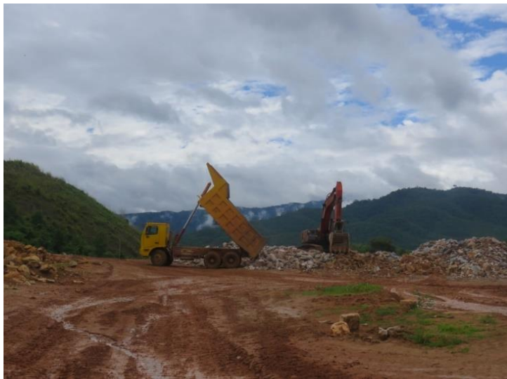
Figure-15: Truck and Bulldozer
